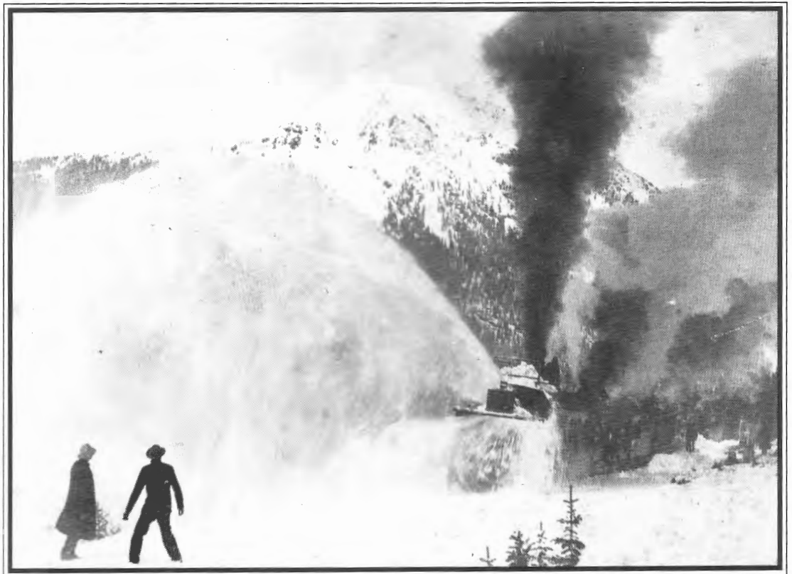
Right: The Leslie Rotary throws a plume of snow some 300 feet as it nears Romley on April 16, 1890, the first day of the South Park Snowplow Trials. Photo by William Henry Jackson, collection of the Colorado Railroad Museum.
