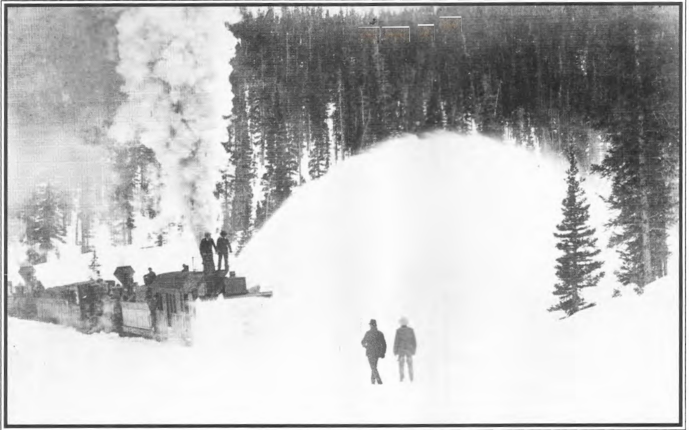
Above: The Leslie Rotary throws snow to the left during the contest. The Jull had difficulty accomplishing this task. Photo by William Henry Jackson, collection of the Colorado Railroad Museum.
