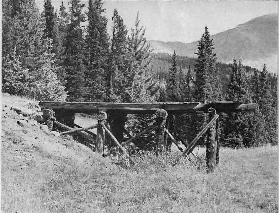
Ore bearing precious metals was once loaded into narrow gauge gondolas from this ramp built near Marshall Pass.
