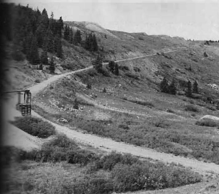
This is the roadbed of the Rio Grande's standard gauge line to the Ibox mining area east of Leadville. The grade was in excess of 4 percent as it climbed up to the mine complex at 11,000. Until it was torn up during World War II, this was the highest standard gauge track in America.
