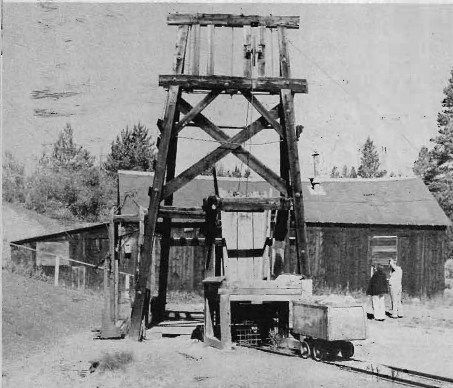
A closeup of the headframe of the Matchless. The bull wheel atop the headframe is probably not the original. Note the cage to the left that was used to transport miners into and out of the mine. The shaft has been covered to prevent anyone from accidentally falling in.
