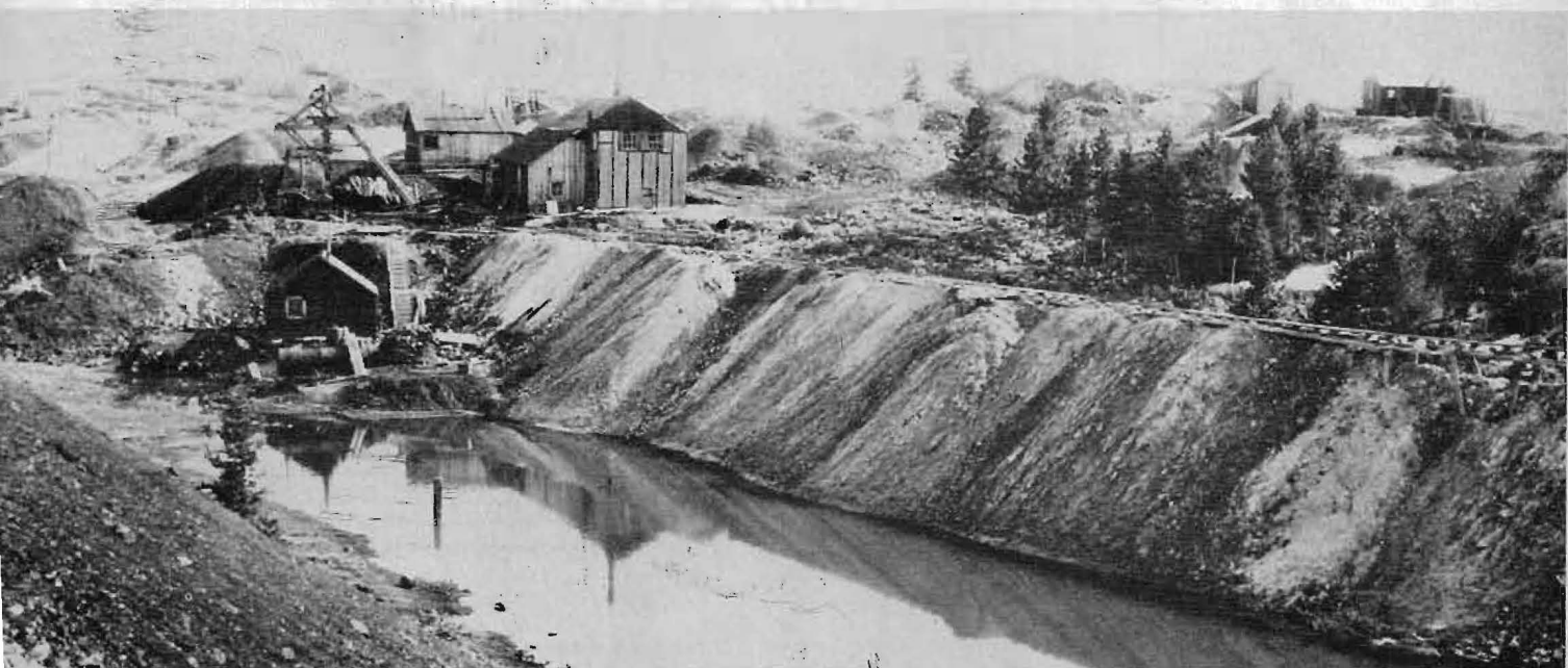
Above: This photo provided by the Colorado Historical Society shows how the Matchless Mine complex looked in 1929. The hoist house had an addition, the headframe was different, and there's a small building near the pond, probably a pump house to clear water out of the mine shaft. On the far side
