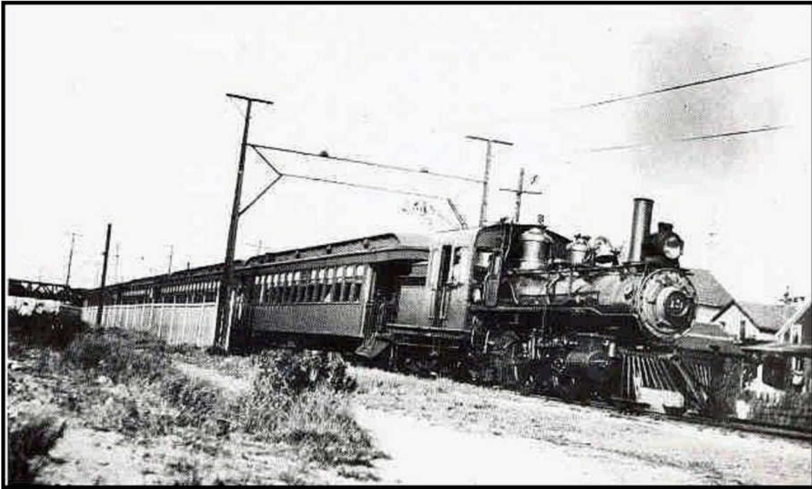
**Figure 34** - Here's Engine No. 19 with her steel cab, caught at work some time between mid to late 1928. She's pulling out of Revere, with the catenary's ominous 600-volt kiss-of-death serpent looming just overhead, so to speak. (RFM)
